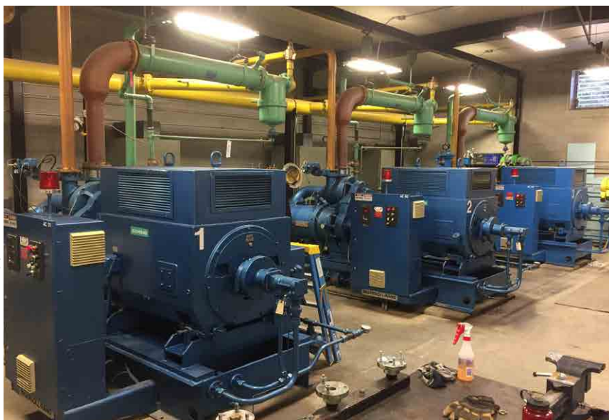
Three main 1,100 HP Centac air compressors
