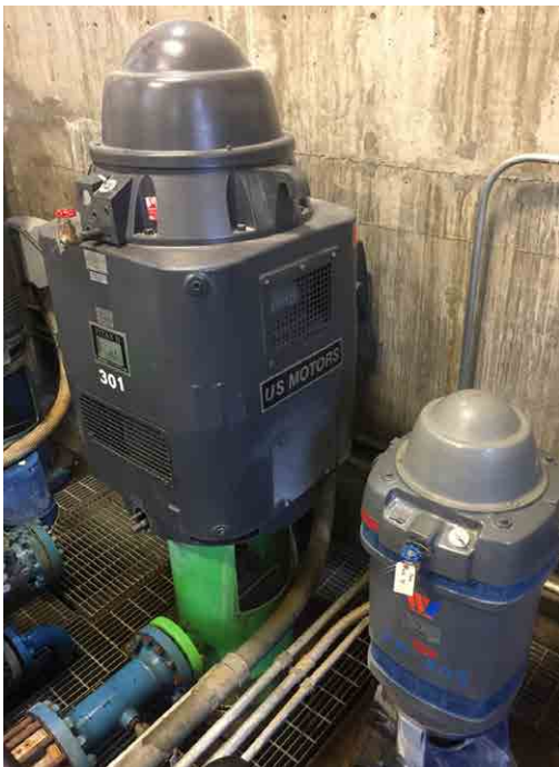
Two pumps - 300 HP and 75 HP
