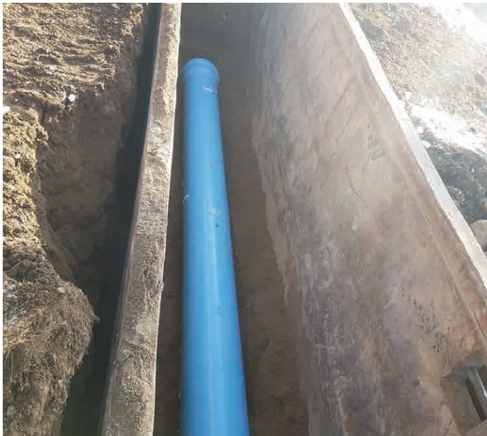
Example of 16-inch PVC in the trench box
