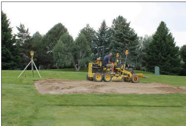
Figure 3: Grading the surface prior to planting.
