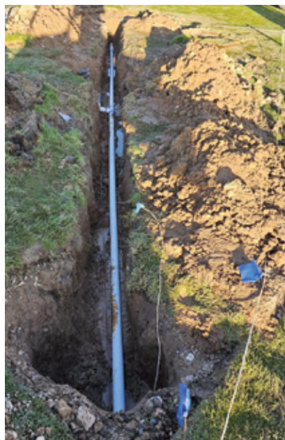
Hole # 5 repair, Redhawk GC
