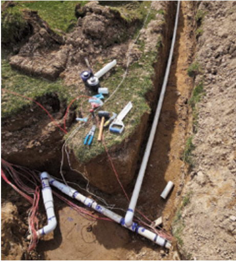
#8 green sprinkler head relocation
